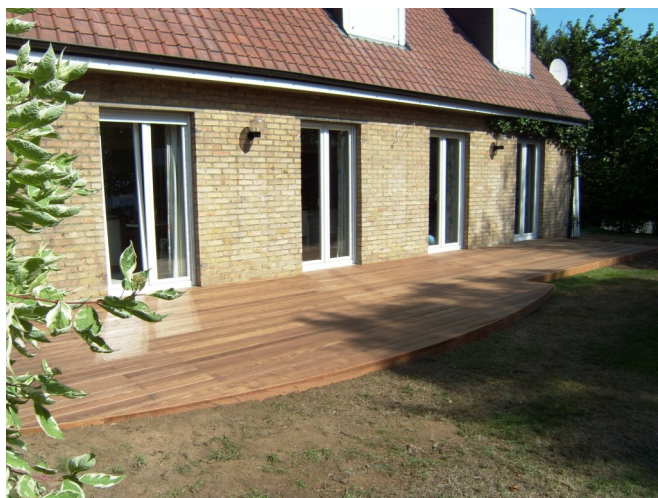
Dimension 26x118, project profile, oiled surface
