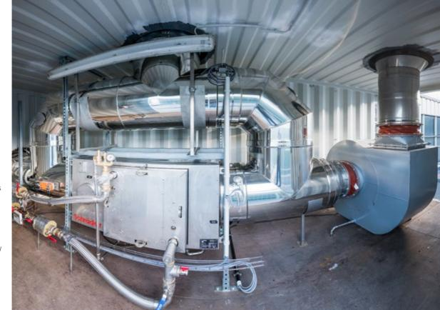
We recover the waste heat from our heat treatment shop using this plant and feed it to our heating system. Using these heat recovery plants at the boiler house, on our air compressors, the ventilation, the hardening plant and the heat treatment shop, we recover over 10 percent of the total energy used at KNIPEX.
